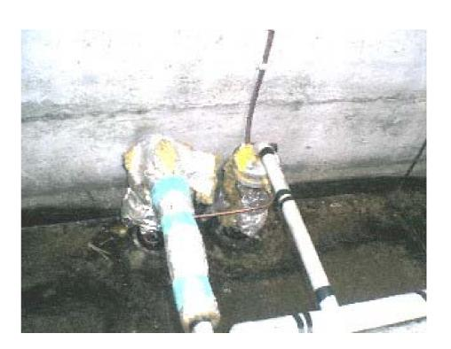
Double shell pipeline with LAG (Leakage indicator) working on the principle of overpressure
